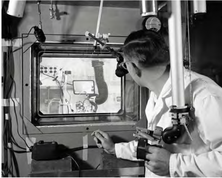
Figure 5-21: Preparation of Pure Pa-233, Alpha Cave
