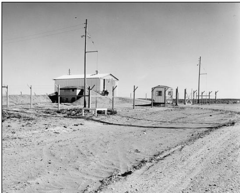
Figure 5-40: The SPERT-I Facility
