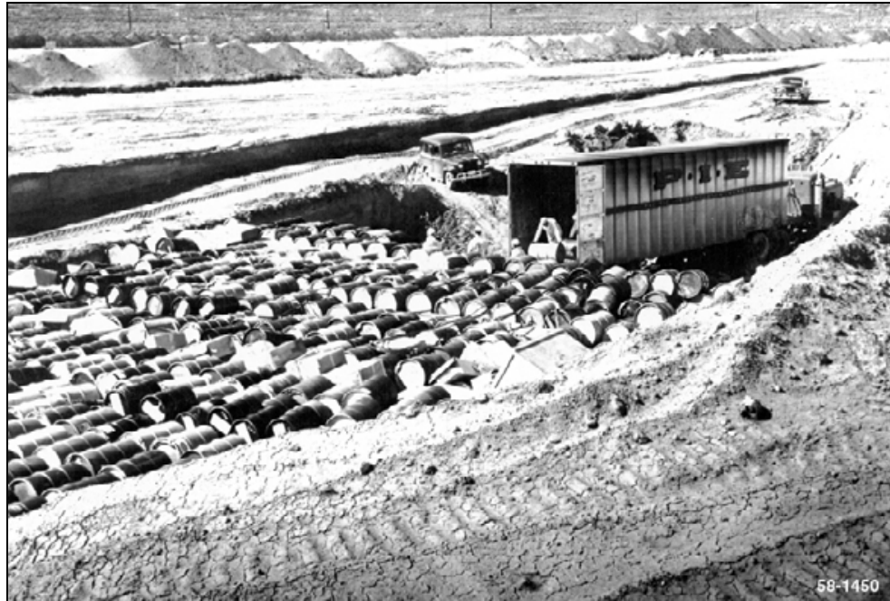
Figure 5-45: Emplacement of Rocky Flats Drums in a Burial Ground Pit in 1958
