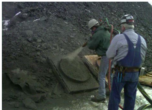
Figure 87. Spraying round panel forms with a dry mix shotcrete.
