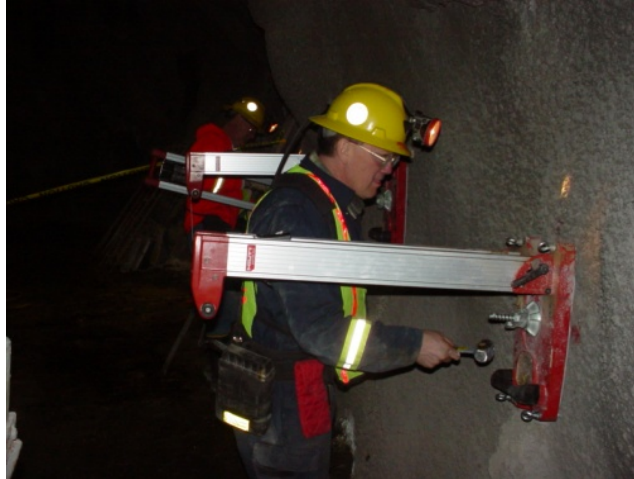
Figure 65. Preparing to remove drill stand and install direct-tension test equipment.
