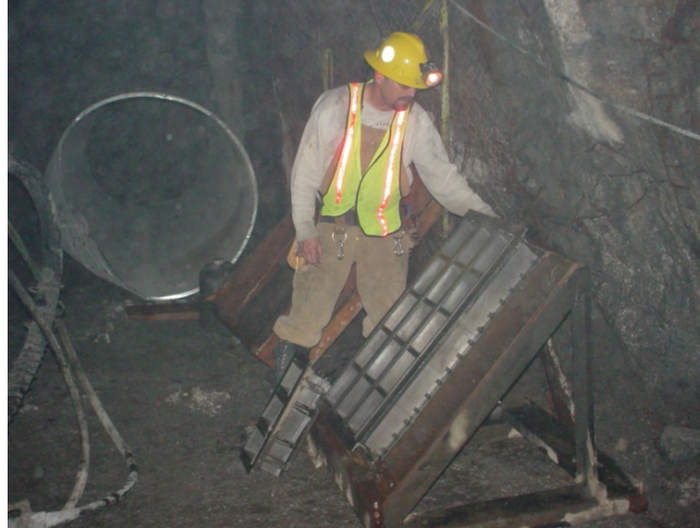
Figure 47. Positioning partial-beam shotcrete molds and containment fixtures prior to shotcreting.
