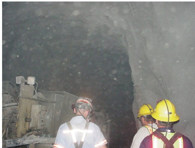
Figure 4. Final in-cycle application of wet mix shotcrete.
