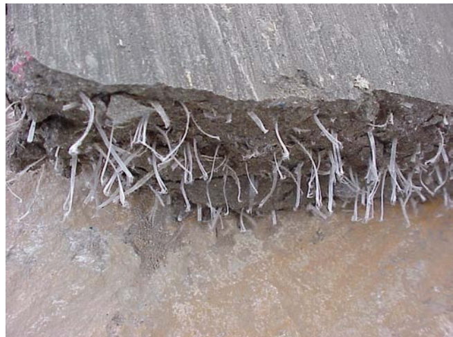
Figure 79. Synthetic macro fibers exposed along the failure surface of round-panel shotcrete sample.
