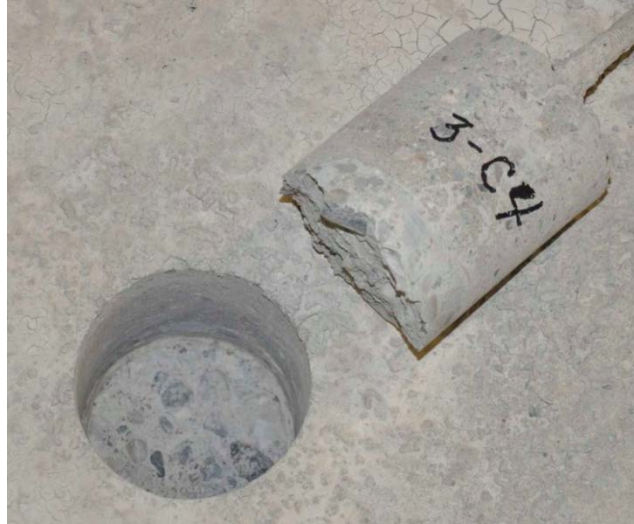
Figure 61. Shotcrete test core and drill hole from a bond strength test with dry mix shotcrete applied to a concrete substrate.
