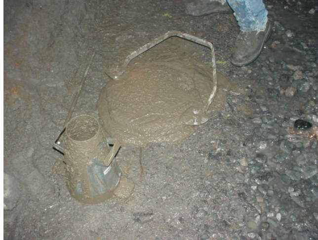
Figure 33. Slump test with wet mix shotcrete showing a 292-mm (11.5-in) slump; typical slump is 100 to 200 mm (4 to 8 in).
