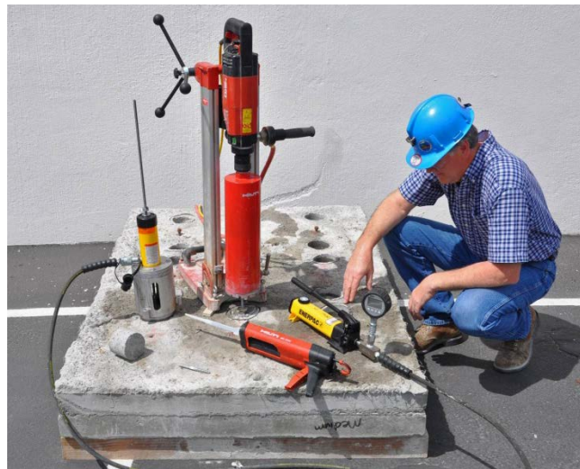
Figure 53. Operation of overcoring and direct-tension test equipment.
