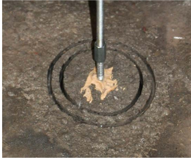
Figure 56. Drill hole configuration with extension rod connected to epoxied stud.
