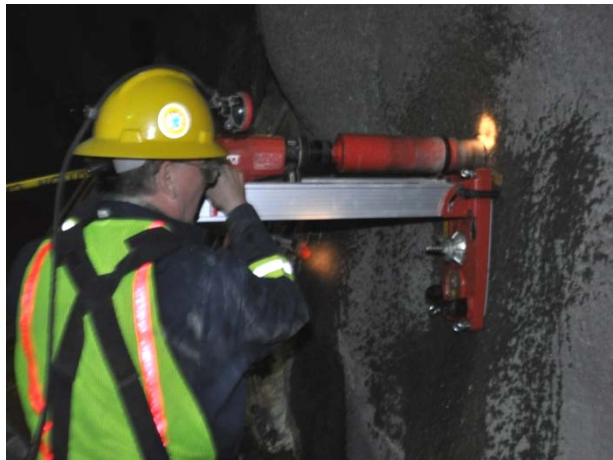
Figure 55. Wet drilling with diamond core bit.
