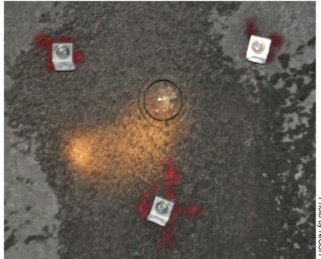
Figure 58. Strap brackets centered around the epoxied stud to anchor the direct-tension test equipment.
