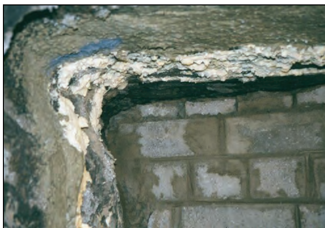
Figure 28.—In background, top of a solid-concrete-block seal showing small cut blocks and mortar filling at the seal top.
