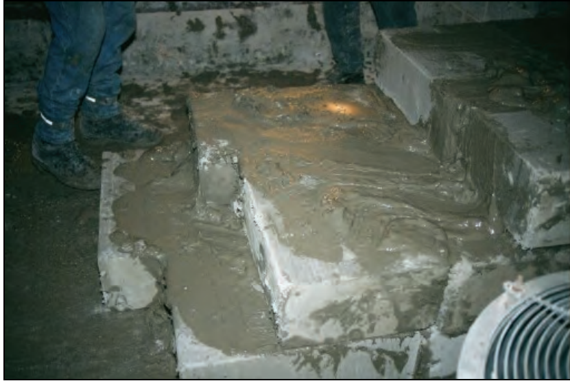
Figure 49.—Construction of a 40-in-thick Omega block seal without hitching and no center pilaster. All surfaces are coated with BlocBond mortar.
