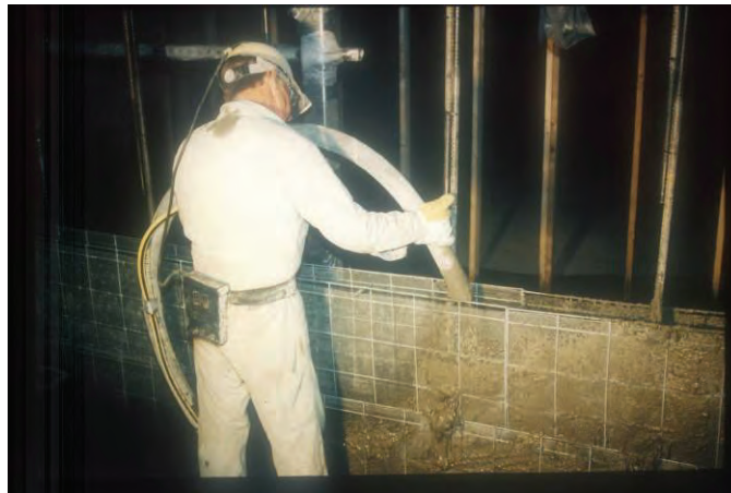
Figure 22.—Meshblock seal under construction showing the lower Meshblocks, the vertical #8 steel reinforcement bars and anchors, and placement of shotcrete.
