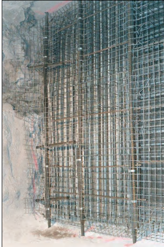
Figure 18.—Insteel 3-D seal under construction showing the rear Insteel panel with Stayform backing, one plane of vertical #8 steel reinforcement bars and anchors, the horizontal #8 steel reinforcement bar anchors, and the horizontal #3 steel reinforcement bars.
