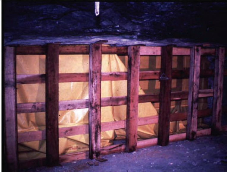
Figure 24.—Formwork for a typical pumpable seal showing the vertical posts, the horizontal boards, and the brattice liner (partially removed).
