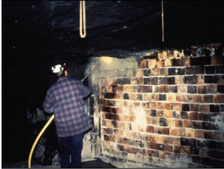
Figure 40.—Construction of a hitched wood-crib-block seal without plywood facing showing the wood crib blocks separated by a rock dust layer, the angle iron hitching around the ribs and floor only, and the final coating with an approved sealant.
