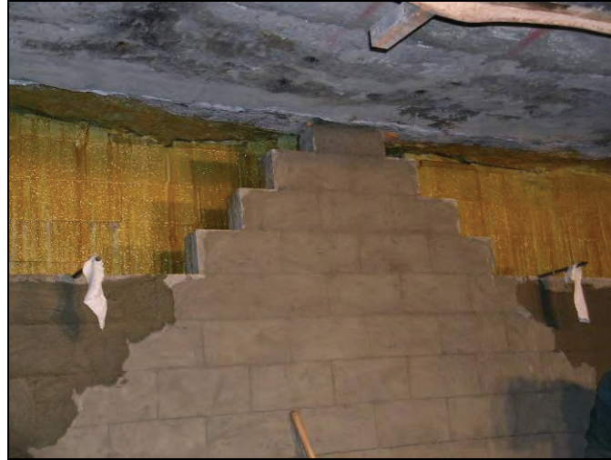
Figure 36.—Polymer and aggregate seal from MICON showing the rear dry-stacked, hollow-core concrete block wall, the partially completed front wall, a polymer coating on the inside surface of the form walls, and an approved sealant on the outside surface of the form wall.
