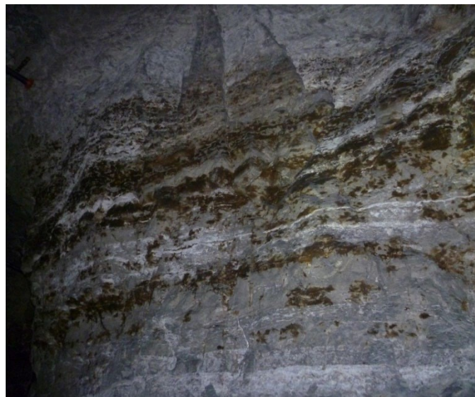
Figure B7. Oil-like residue on cavern wall. Photo by NIOSH.
