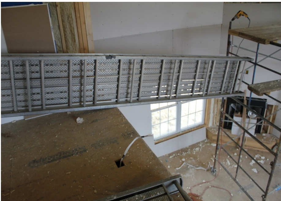
Figure 2. Position of the plank after it had flipped onto its side. Photo taken from loft area
