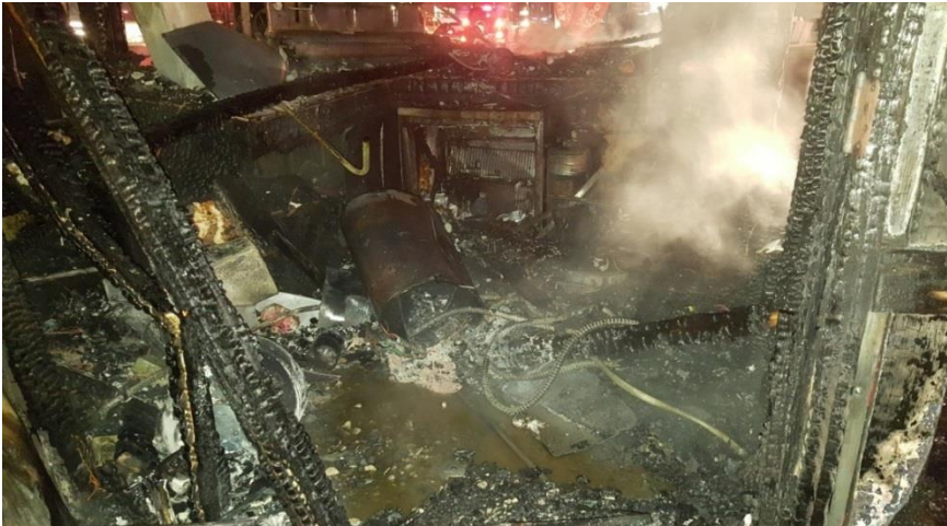
Photo 2: The coffee stand interior after the fire.
