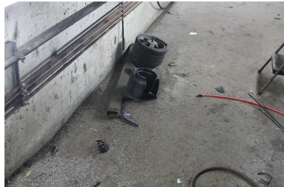
Figure 1. Left side air spring after the explosion.
