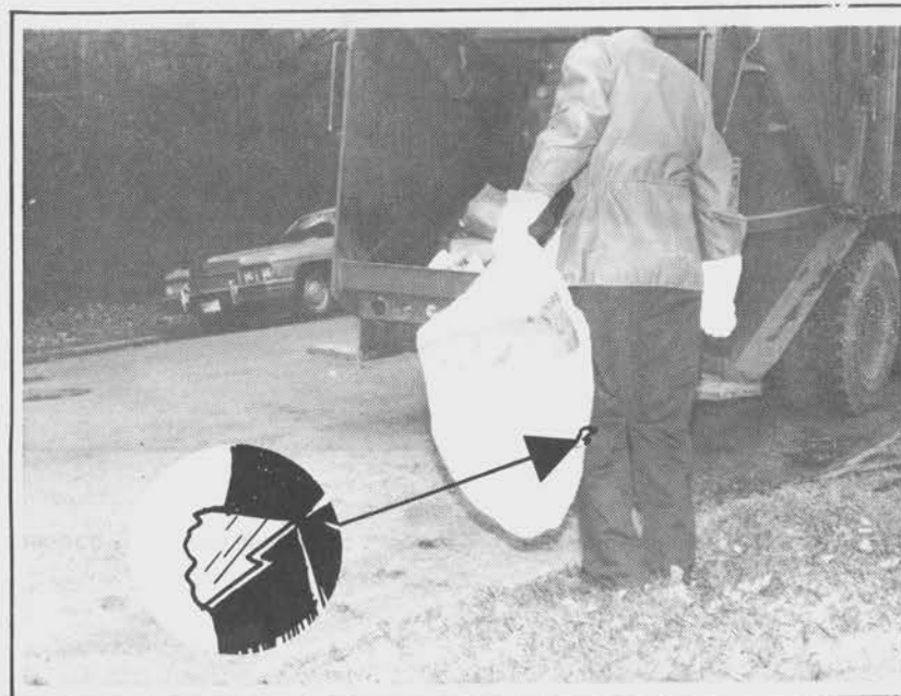
Figure 54. Keep bag clear of leg to prevent cuts from protruding glass or metal.
