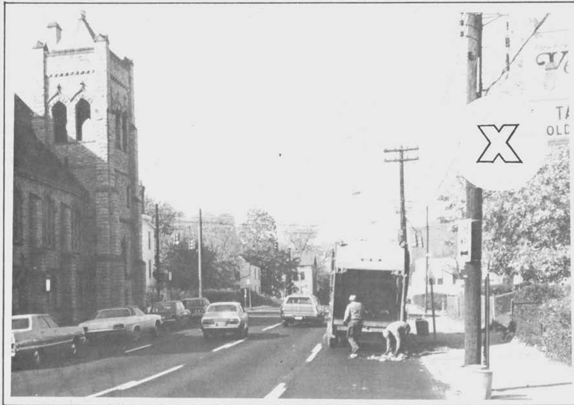
Figure 100. Truck should have carried broom and shovel for popouts.
