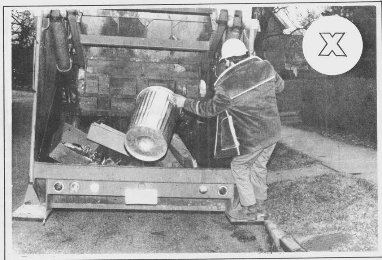
Figure 37. Don't lift or load from riding step.
