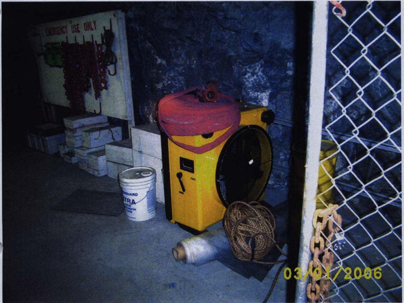
Additional emergency supplies stored in permanent refuge chambers
